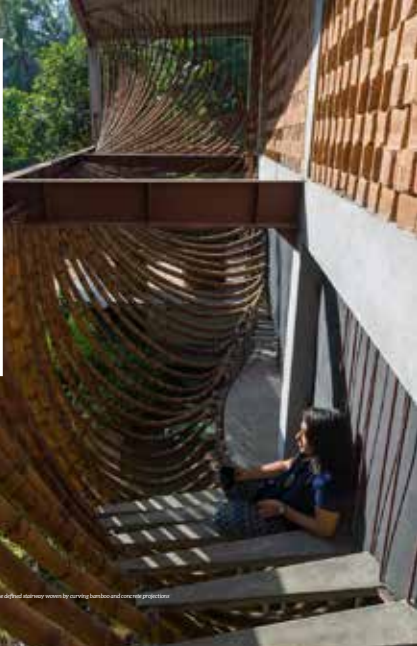
The defied stairway woven by curving bamboo and concrete structure
