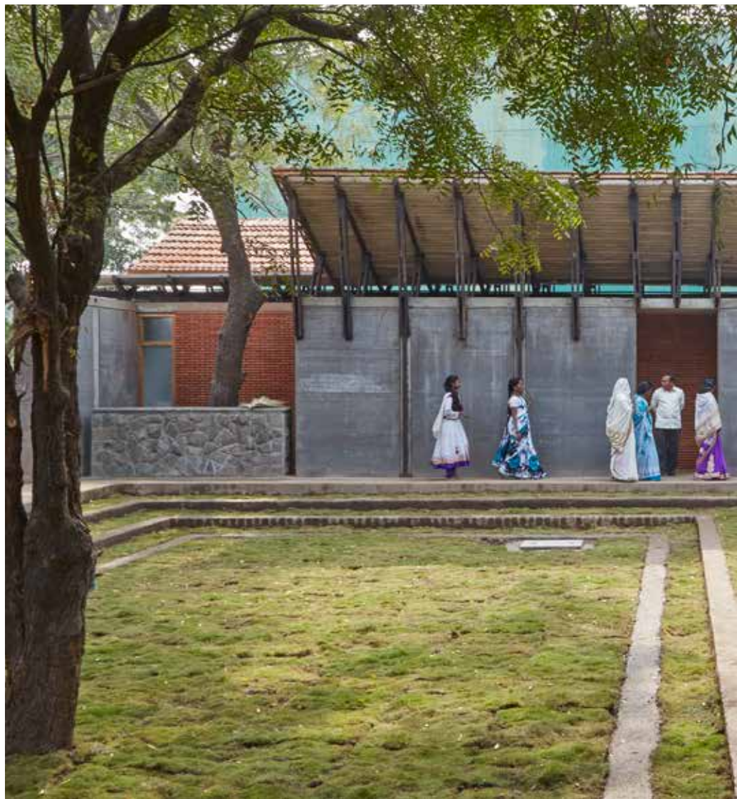
The basal stone dust rammed earth walls supporting the 'butterfly' roof
