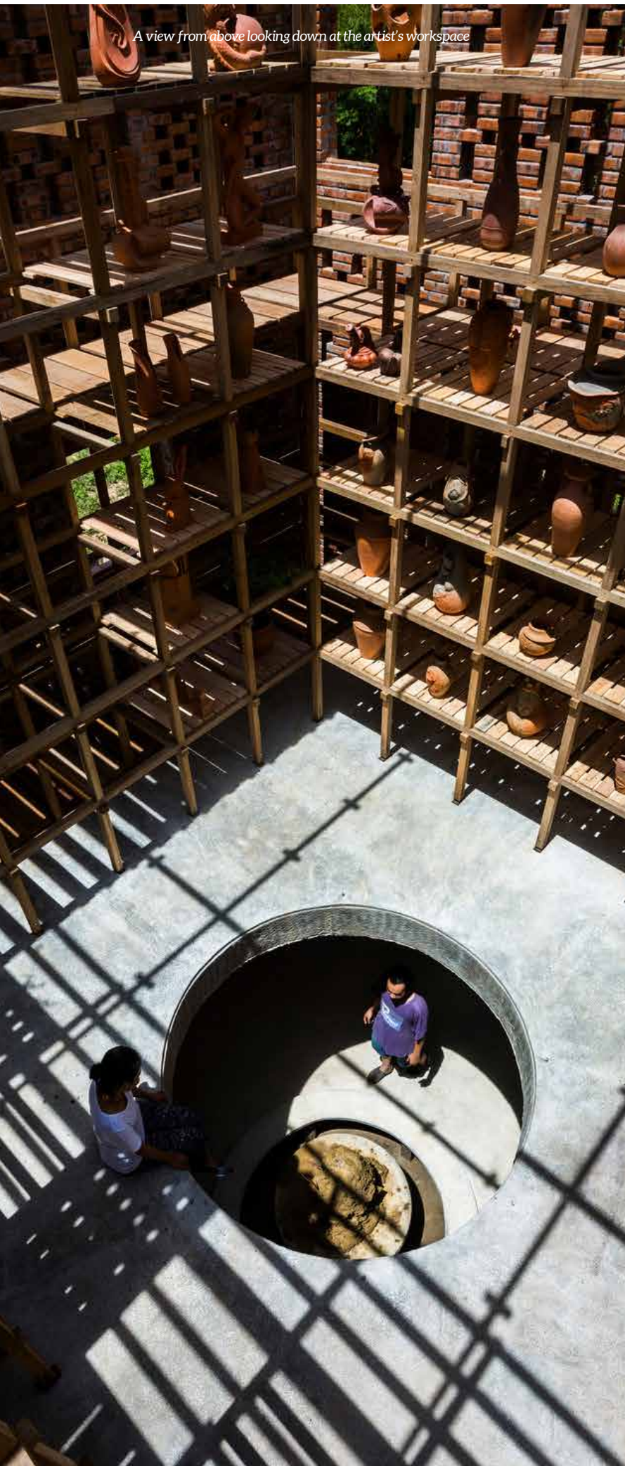
A permeable pattern of brick that forms the skin of the studio
