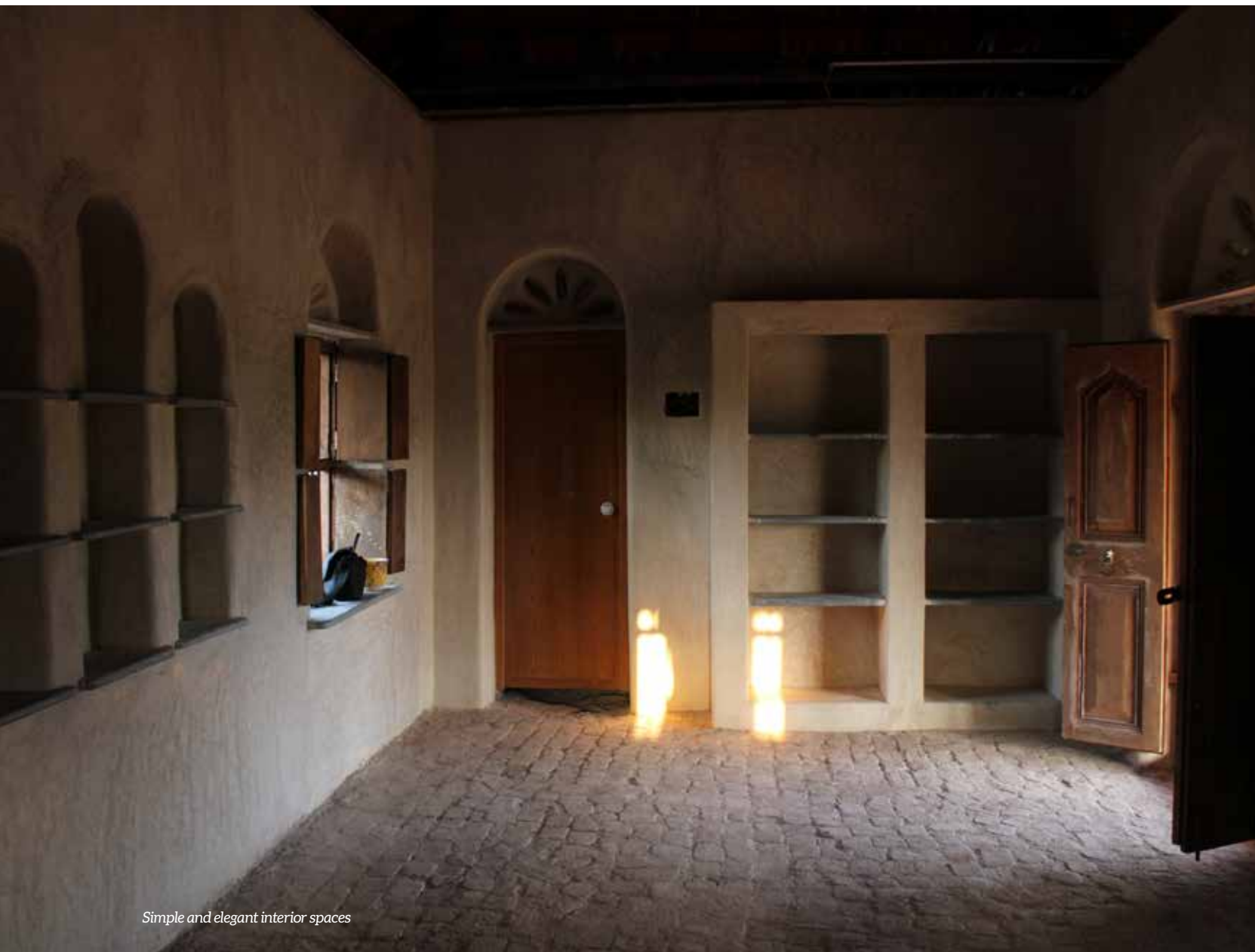
Slabs pierced into the adobe walls
