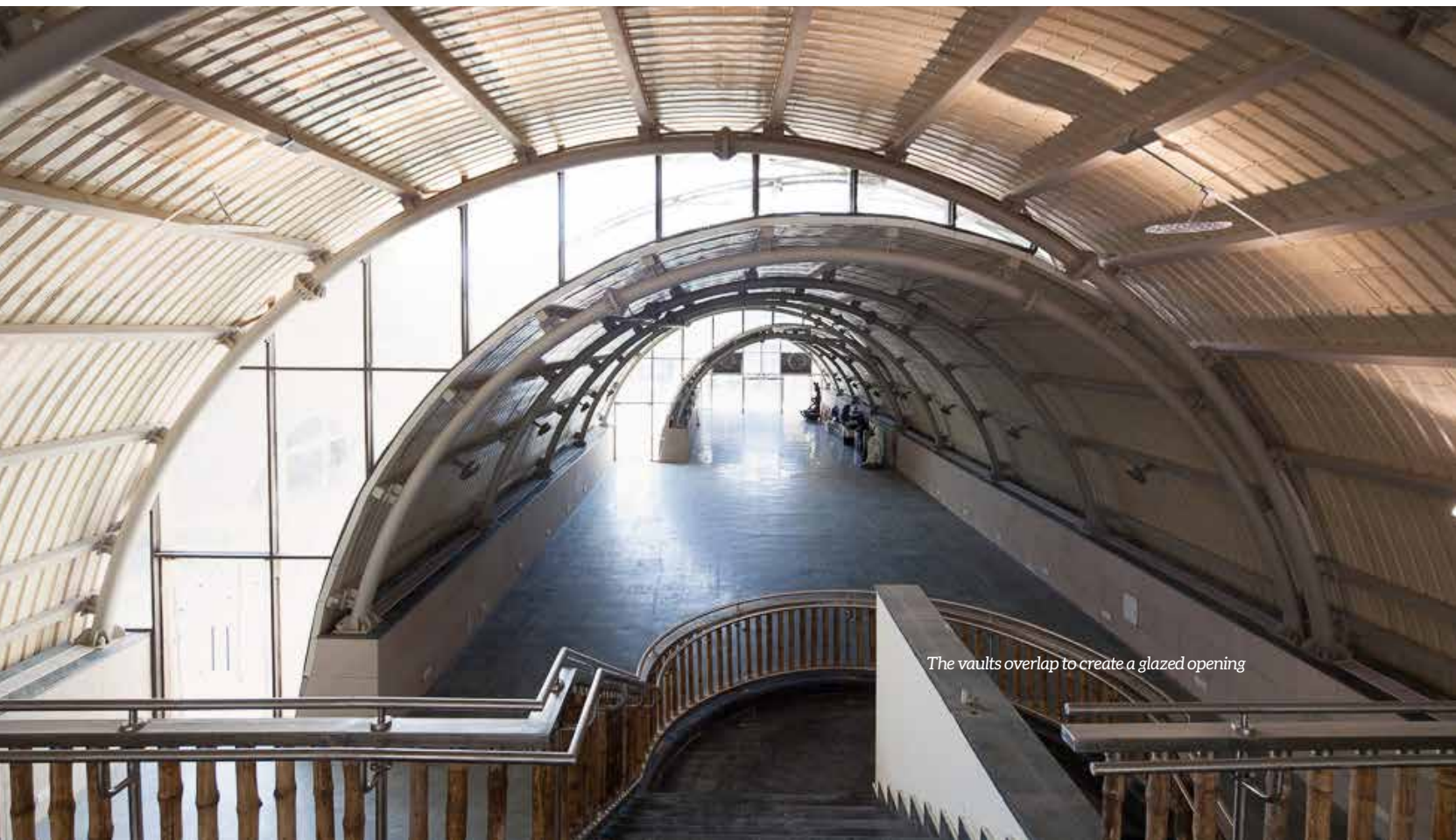
Barrel vaulted structures
