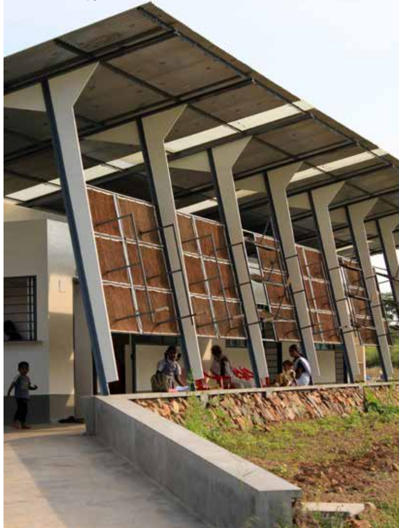
The rubble masonry plinth wall that resonates with the local built character
